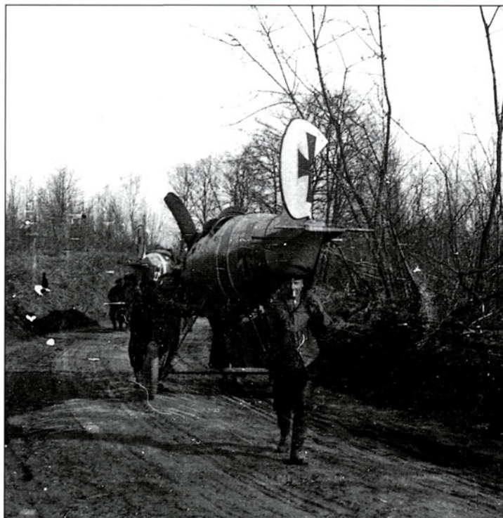
Jasta 'Boelcke' mechanics manhandle two Albatros D V fuselages down a road during the winter of 1917/18 in this interesting photograph from Wilhelm Papenmeyer's collection. The nearest aircraft displays the black and white tail section of the Staffel and the thin black border on the rudder and tailskid fin (Papenmeyer album)
